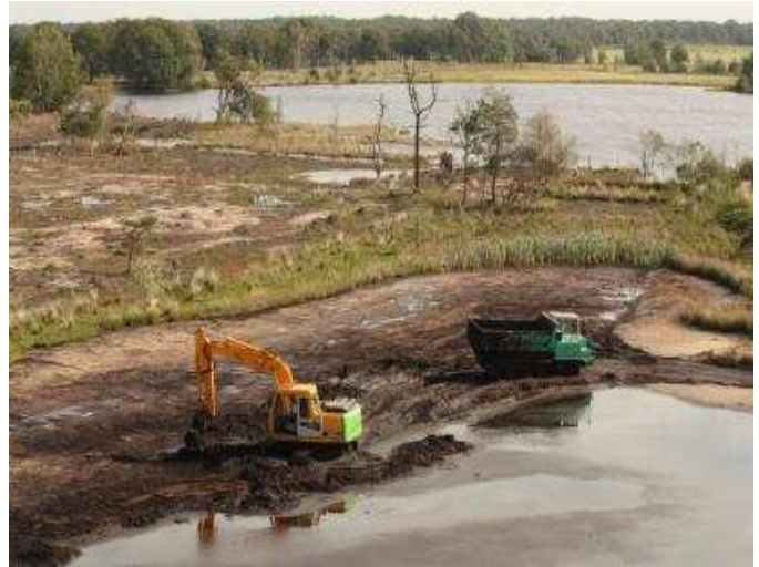
Sludge removal at Kleine Klotterwaard in 2011 Photo: Mario De Block
