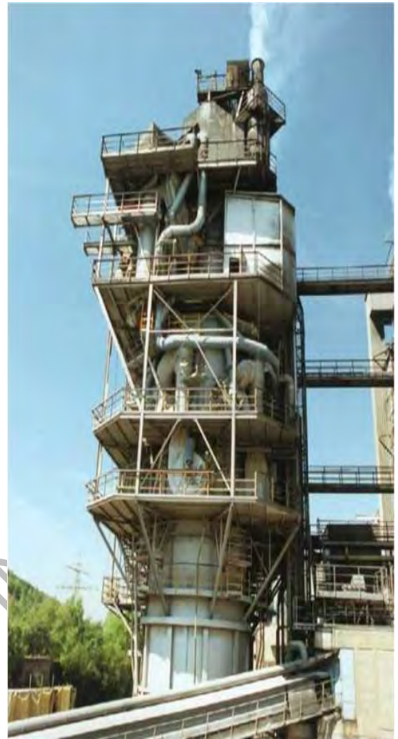
Figure 2.26: Example of an annular shaft kiln used in lime manufacture1
