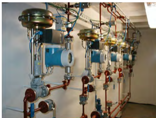
Figure 6.28: Measuring and dosing station with pneumatic valves
