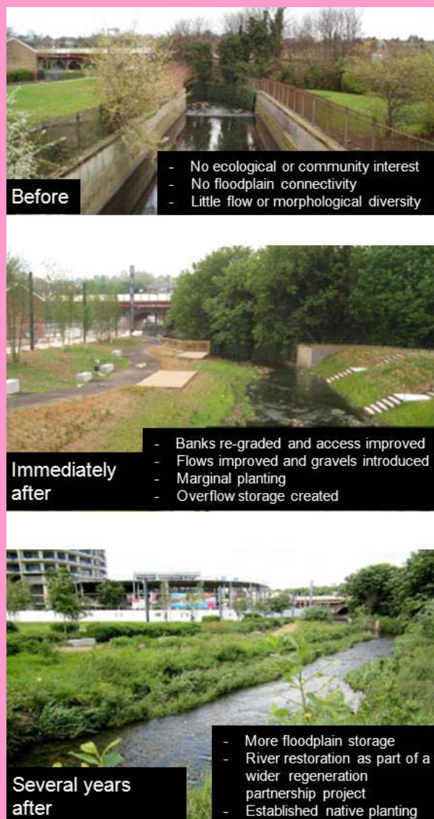
Figure 4.3 River Ravensbourne in south London , before and after its restoration
