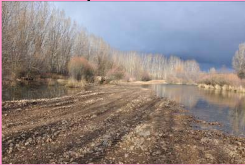
Works recently completed
