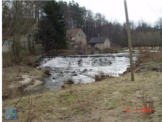
Figure 5.6 River prior to weir removal
