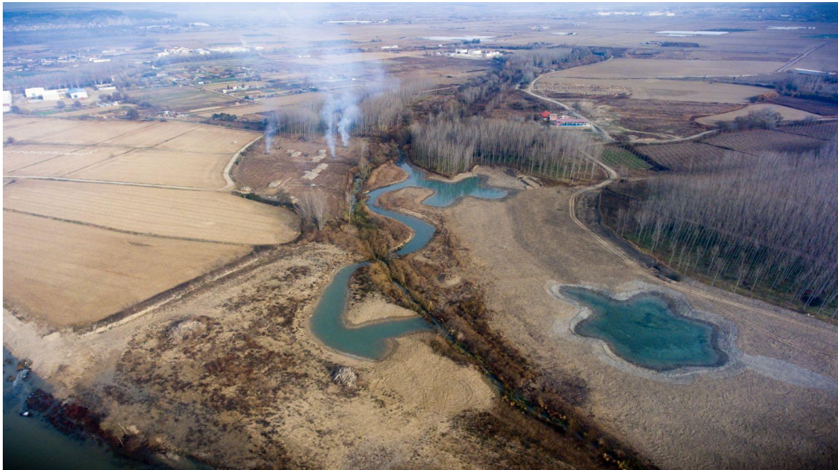
Figure 5.4 Panoramic view of the area and detail of the new wetlands created
