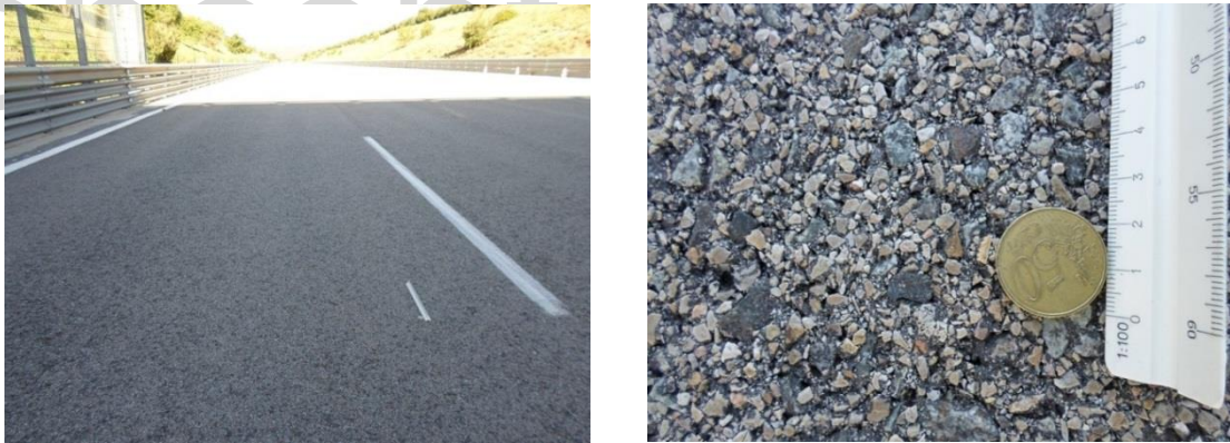
Figure 38: The high-speed circuit and associated asphalt structure
