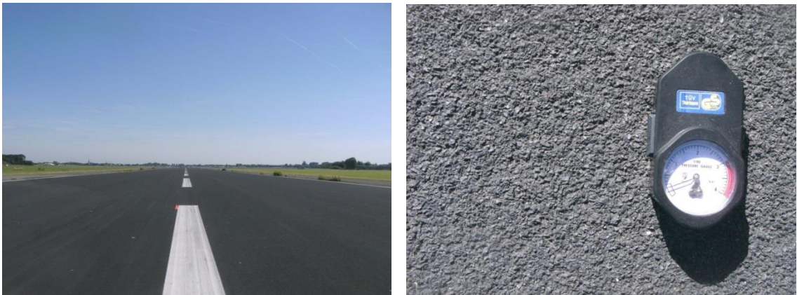
Figure 36: The air-strip and asphalt structure at air base Valkenburg
