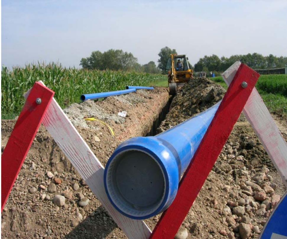
Figure 5.27 On-site Pipe storage
