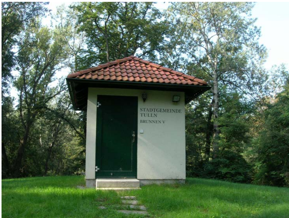
Figure 5.10 Control Measures - spring
