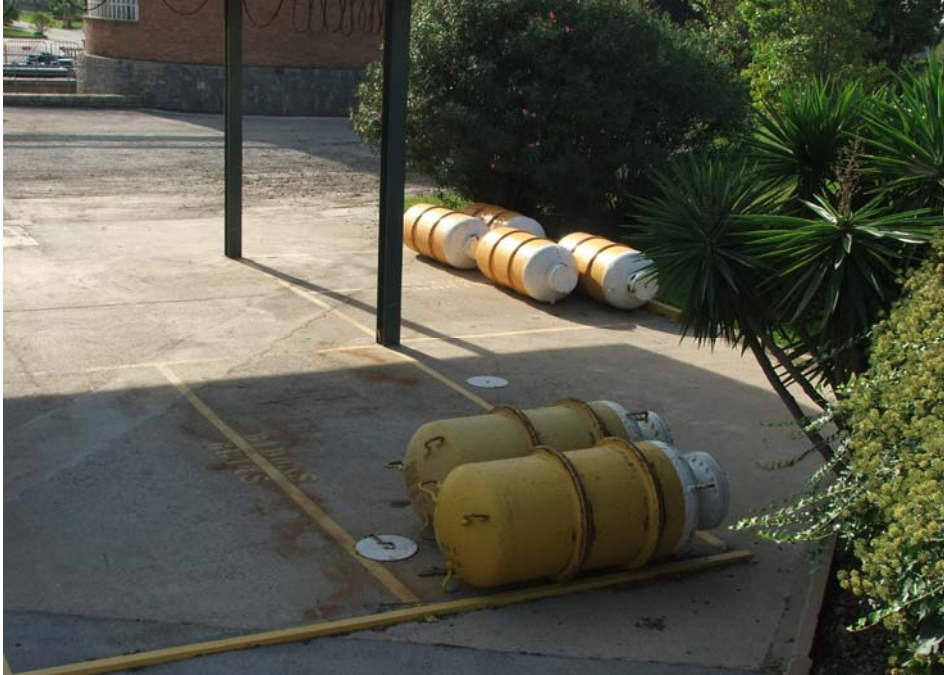
Figure 5.5 Storage of hazardous chemicals
