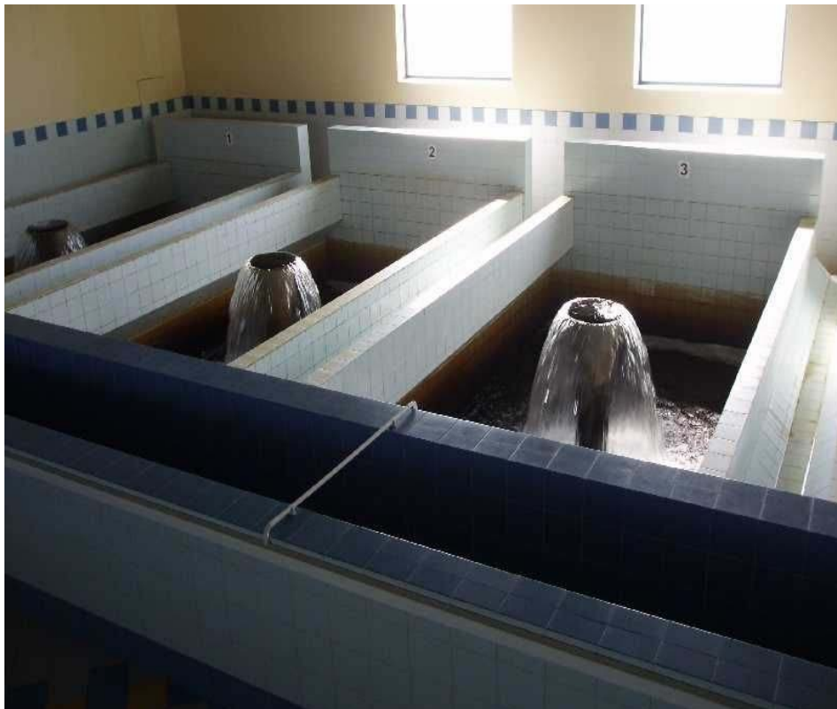
Figure 5.20 Placement of filters in closed building protects from bird intrusions and stabilizes temperature (Klaipeda)
