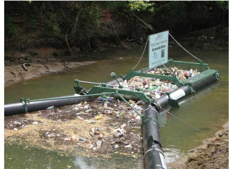
Bandalong Litter Trap in Watts Branch in Washington, DC after one rain event http://stormwatersystems.com/bandalong-litter-trap-installations/
