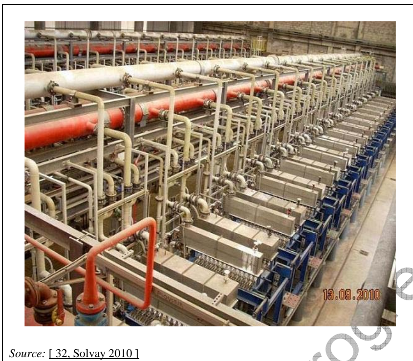
Figure 2.11: View of a membrane cell room equipped with monopolar electrolyzers
