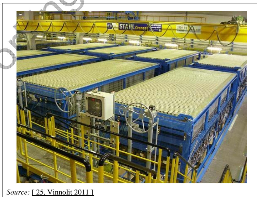
Figure 2.10: View of a membrane cell room equipped with bipolar electrolyzers
