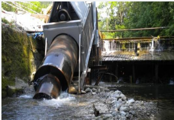
Installing fish-friendly turbines
