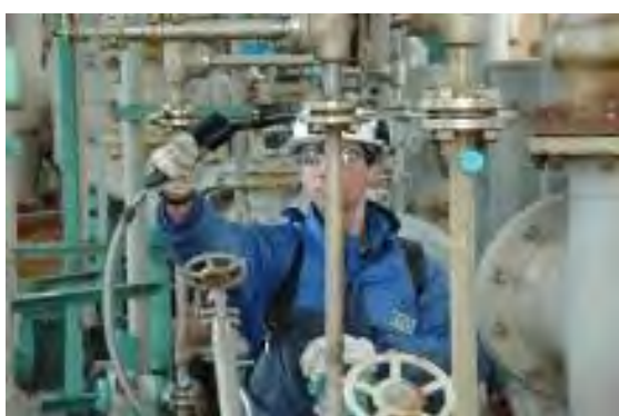
Figure 3.37: Leak concentration measurement
