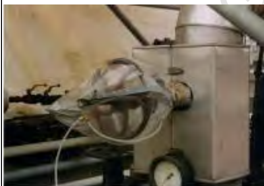
Figure 3.38: Bagging of a leaking valve
