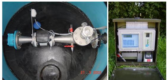
Figure 13 – District meter manhole (left) and installation cabinet for district meter.
