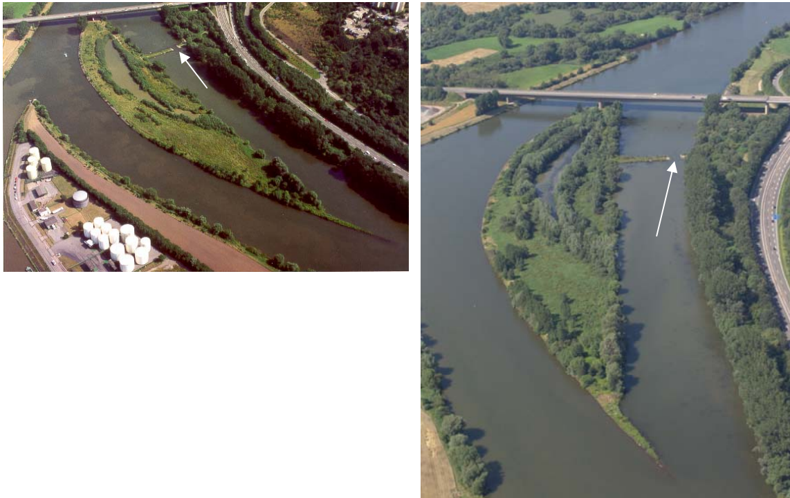
Figure 1: Hahnenwehr floodway (Photo of 1999 left, photo of 2004 right-arrow marks the interrupted courseway).
