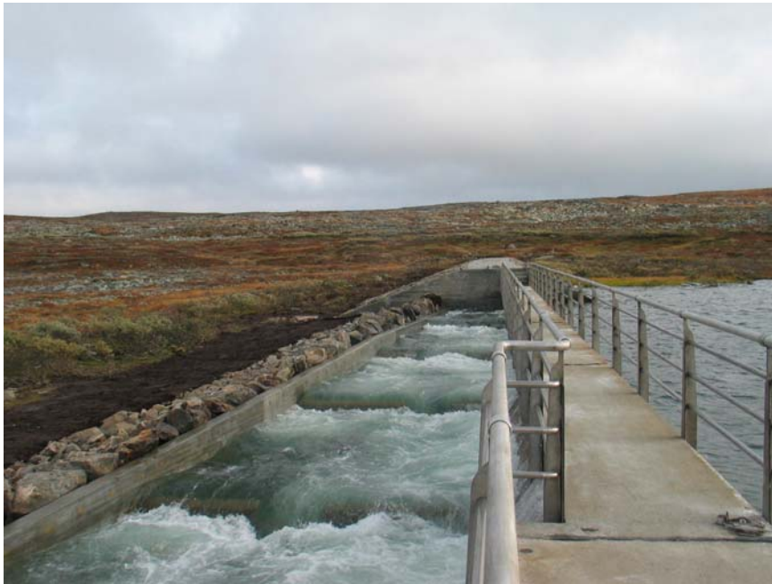
Figure 2: New fish pass at the dam of the Halnefjorden reservoir.
