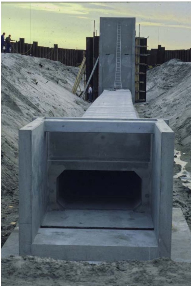
Figure 1: Culvert in the dyke between the Ems-Dollart.
