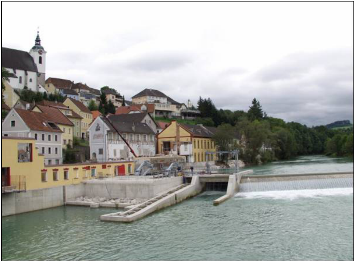
Figure 1: New Steinbach HPP.
