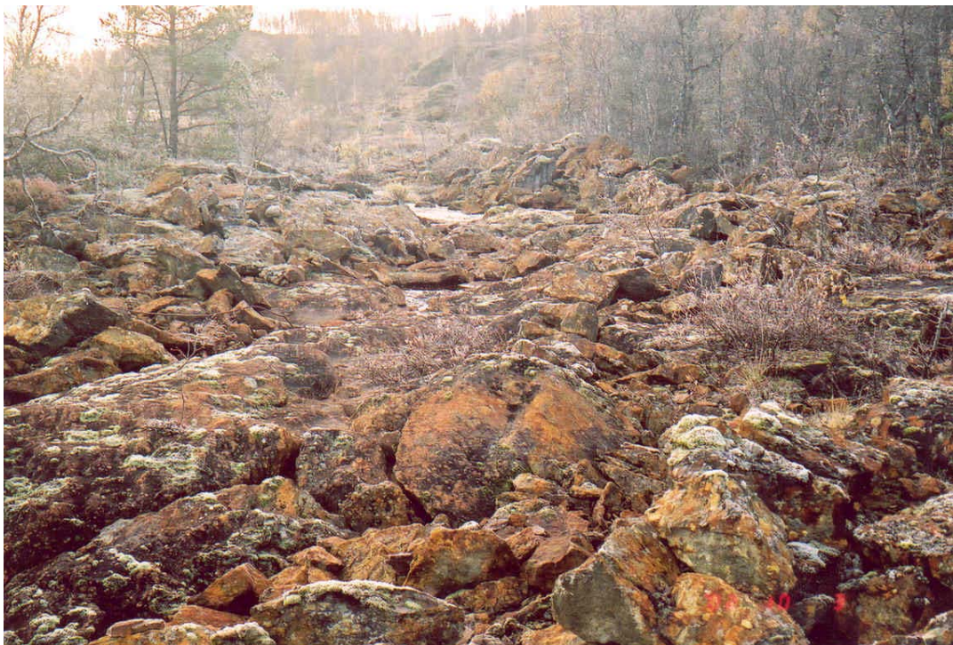
Figure 3: River stretch in the upper part before mitigation. A low amount of water is flowing and the stone embankments are lying along the canalized profile. Done in 1922.
