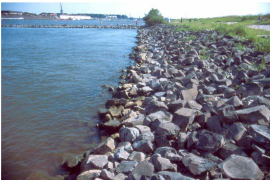
Figure 1: River Rhine at Duisburg, bank reinforcement (stone filling).
