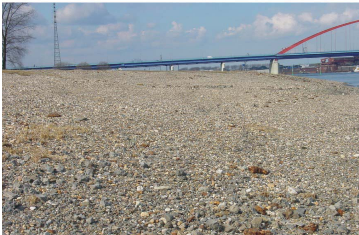
Figure 2: River Rhine at Duisburg after morphological improvement; structures will be created by the next floods and should be maintained
