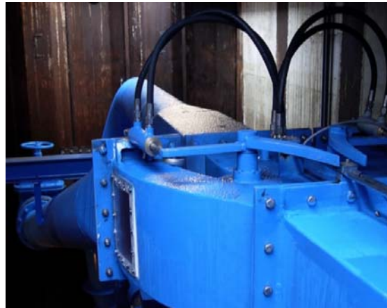
Figure 3: The Venturi at Waterboard Hunze & Aa's.
