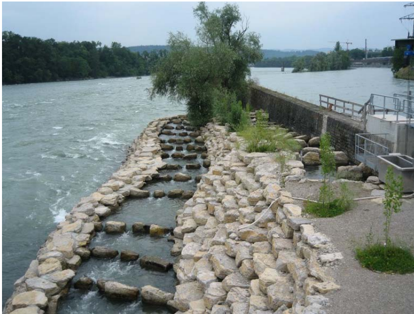
Figure 3: The 150 m long pool fish pass at the new weir.
