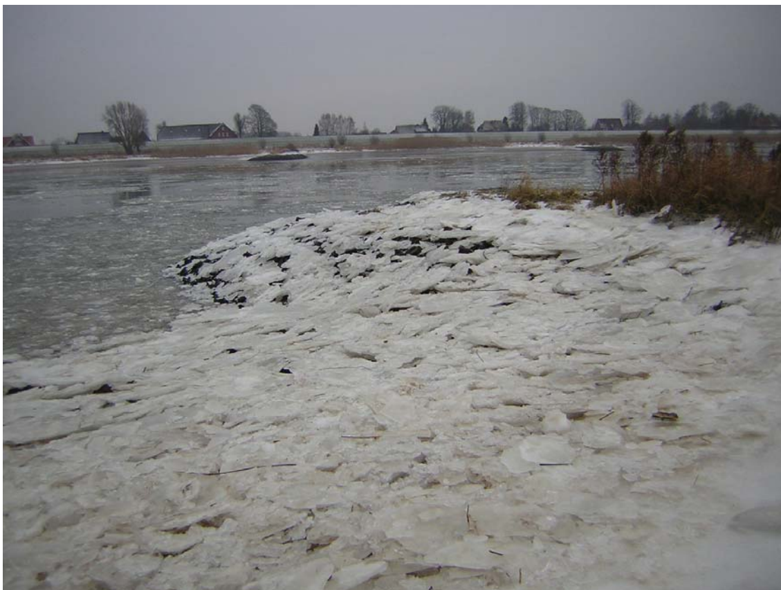
Figure 2: Southern end of the reconstructed revetment. The difference in the design of the bank profile can be noticed clearly.
