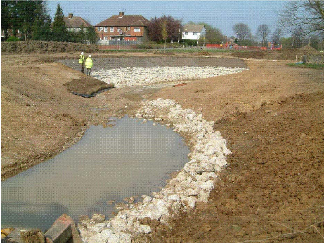
Figure 1: Status during construction.
