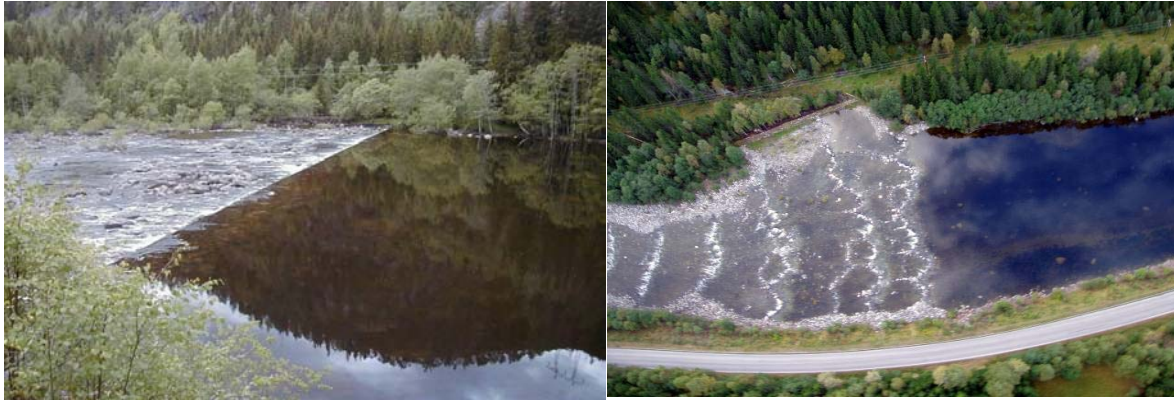
Figure 2: Section of part of the river before (left) and after new weir constructions (right - water flow from right to left) (Photo: NLB).
