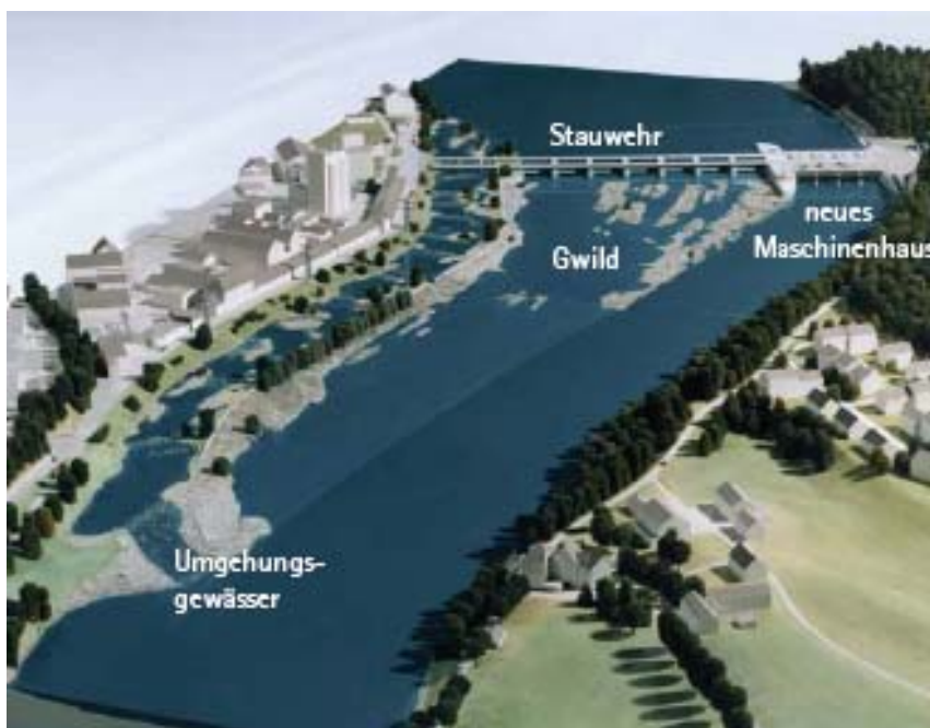
Figure 2: Hydropower plant of the replacement construction (completion in 2011)
