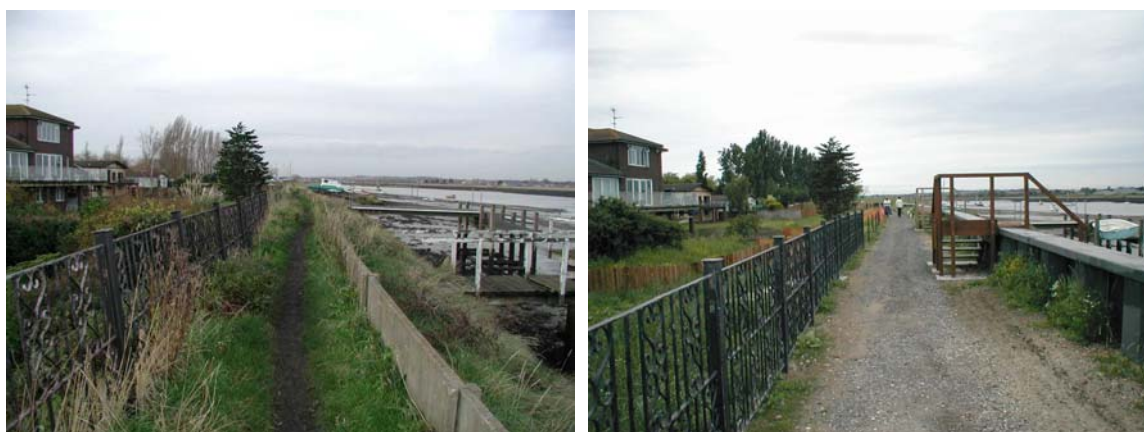
Figure 1: Defences which required improvement (left) and new defences at end of works (right).
