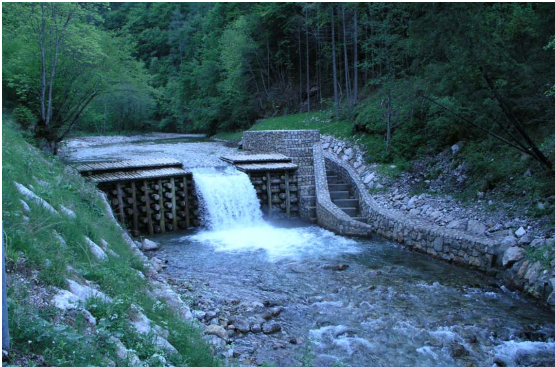
Figure 2: Dam on the Kokra River after restoration works, situation in 2006.
