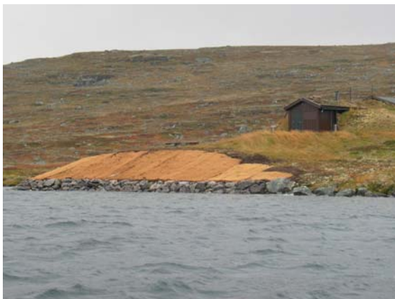
Figure 3: Coconut matting in the littoral zone of the Halnefjorden reservoir.
