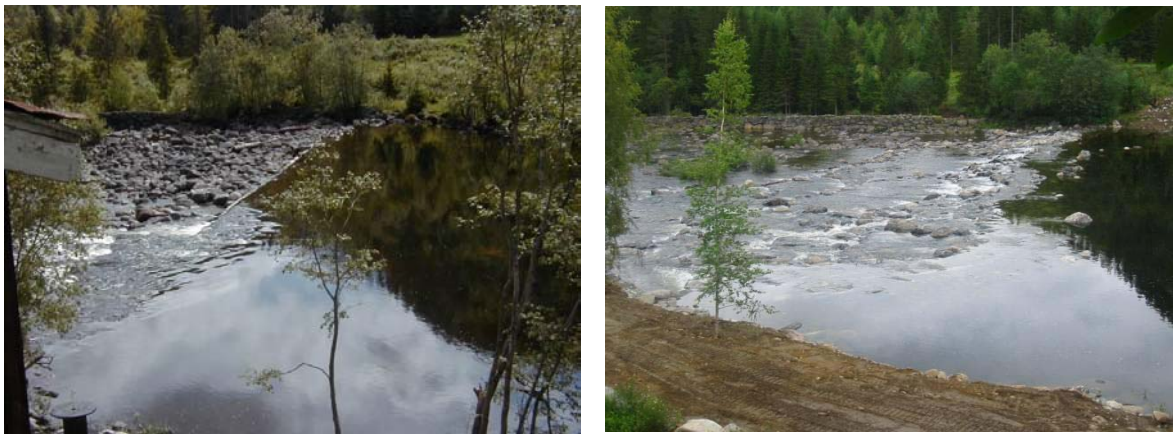
Figure 3: Man-made weir in part of the river before (left) and after weir reconstruction (right). Water flow from right to left. (Photo: NLB)
