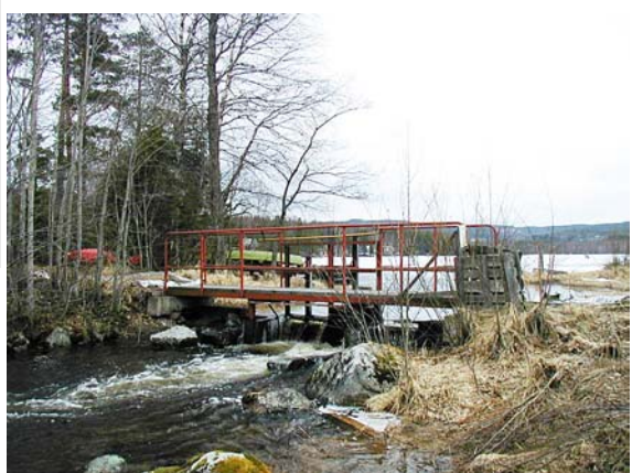
Figure 1: The pictures show the outlet of Storsjön before (to the left) and after (to the right) reconstruction of the natural outlet of the lake. The lake is situated in the upper part of the river basin drainage area. The drainage area of the lake is 33 km 2 and the mean flow in the outlet is 0.4 m 2 /s.
