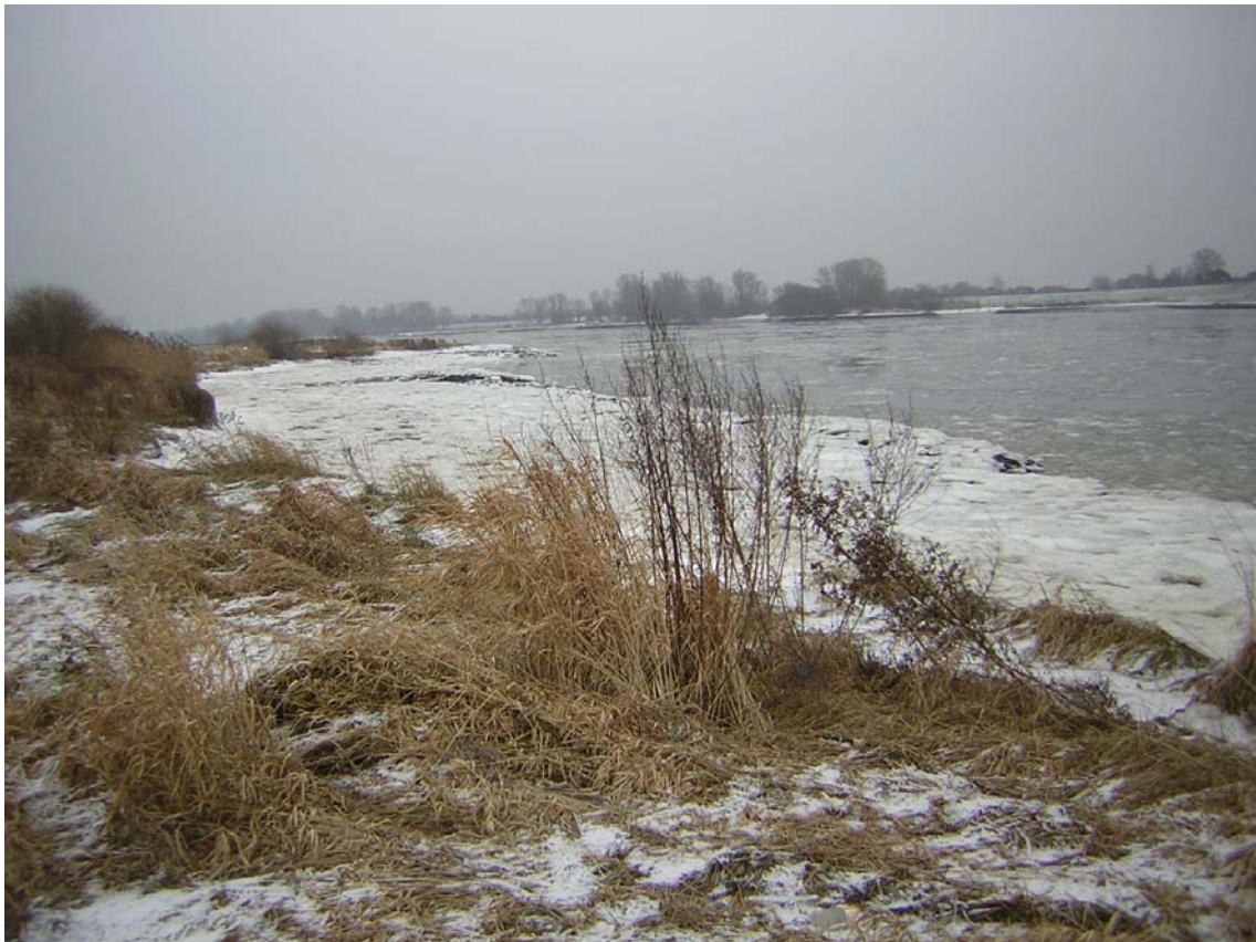
Figure 1: View of a reconstructed section of the river bank (length of section: about 100 m), January 2006 at low tide. The iced marks the zone of the bank which is flooded at high tide.
