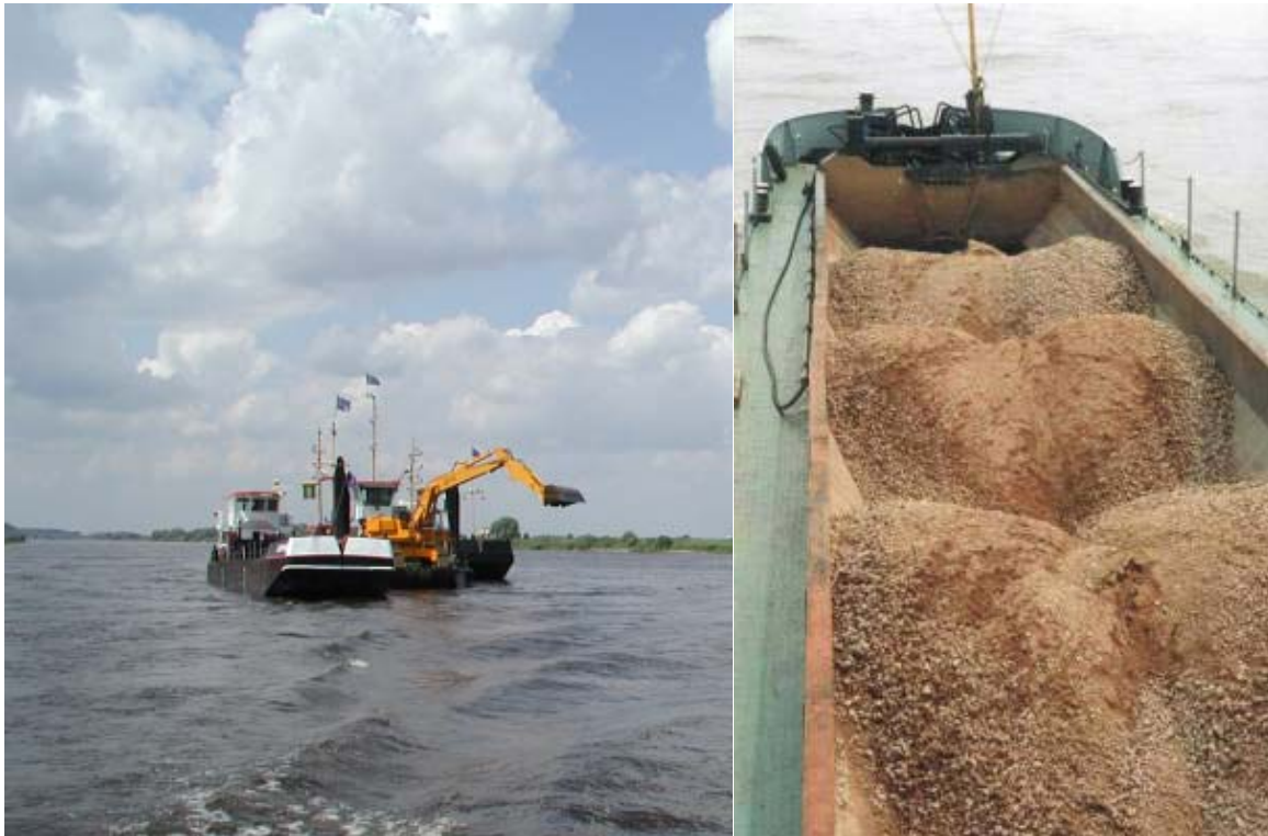
Figure 2: Dredging and dumping of additional bed load into the "Erosionsstrecke" of the Elbe River.
